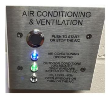
The inbuilt conditioning unit controls shall control the temperature based on the room heat loads. The air conditioning systems shall be interfaced with the Mechanical controller (MCP) for the Communal Building, which will manage the on/off and status indication of the air conditioning systems.
